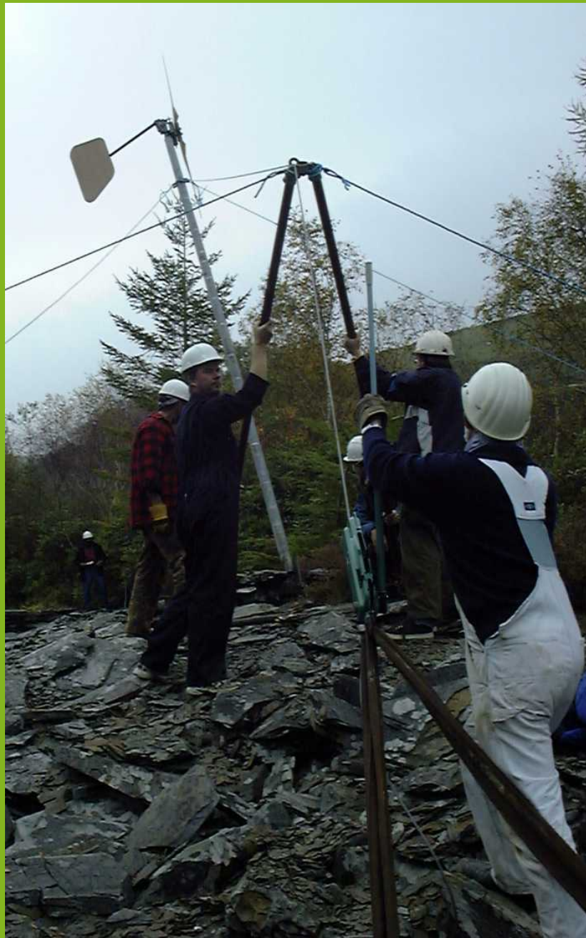
Erection on site at CAT.
