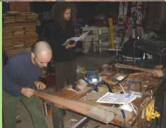
tapering the trailing edge
