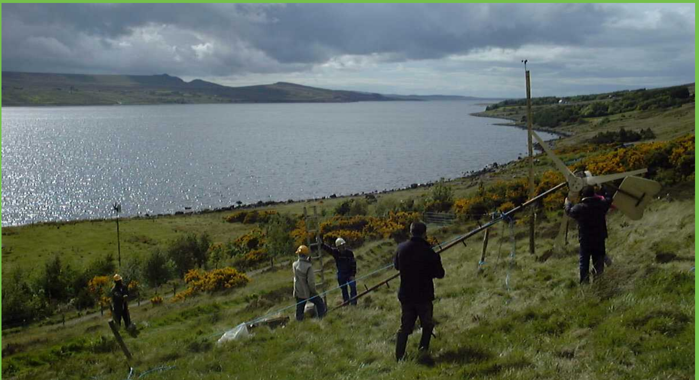
Pic 33: We were all looking - somewhat in awe - at the wind turbine we started building from scratch just 5 days ago actually generating electricity. What a rewarding moment!(We had an anemometer to check the windspeed. It was mostly around 3-5 m/s (7-11 mph) Output was around 20-100 watts. Hugh)
