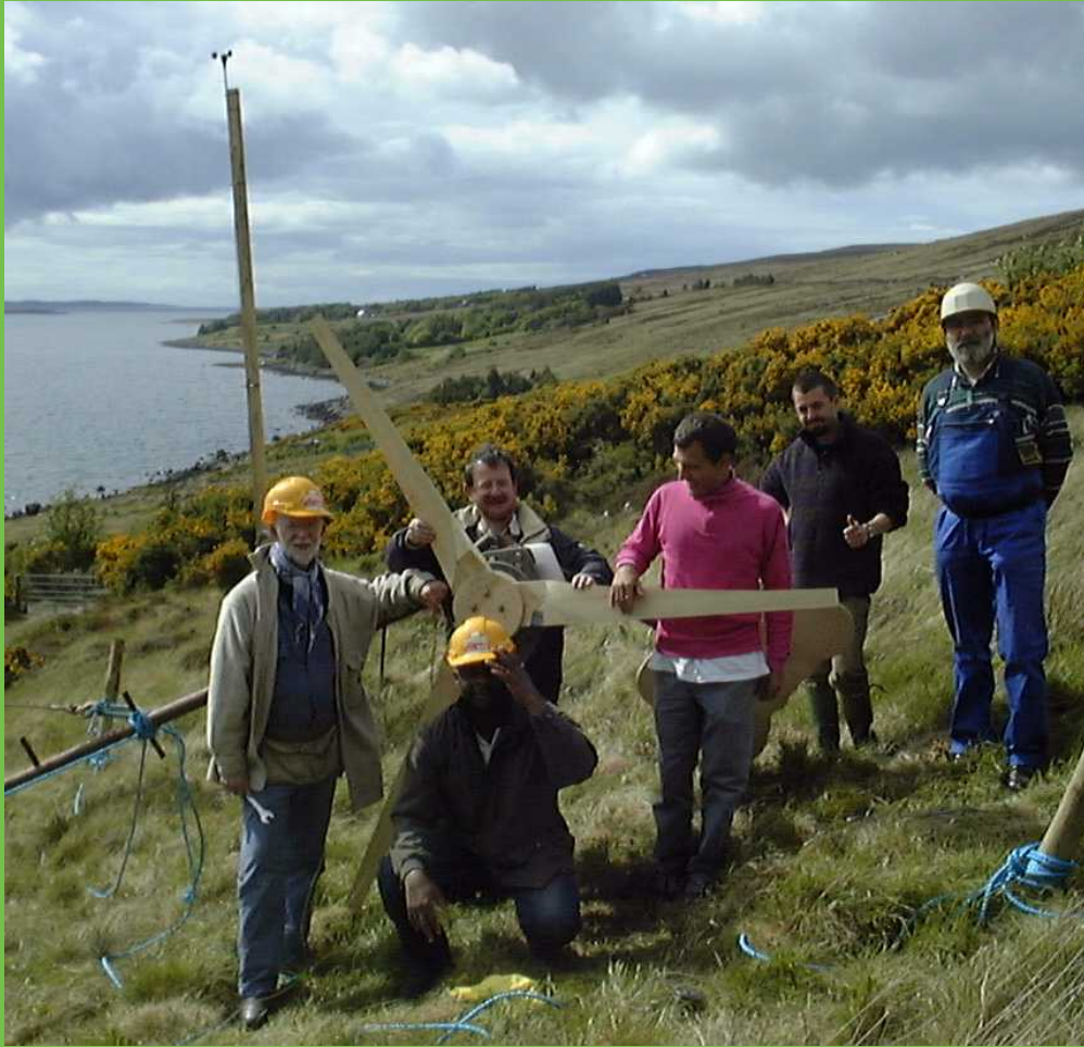
Pic 32: Julius Tangka is operating the winch while John and Uwe use the ladder to guide the cable. Note that the tail is in full furling position. Some rain clouds were approaching and we hoped to see some gusts, but....
