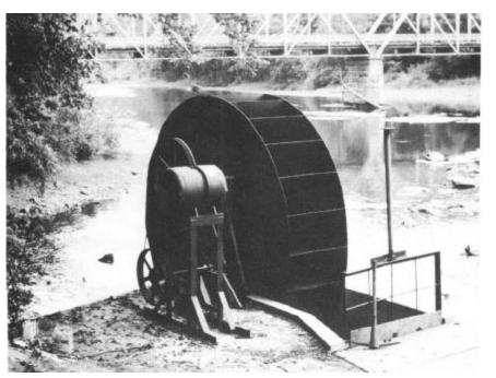
The undershop wheel from the previous page, plus attached generator, installed.
