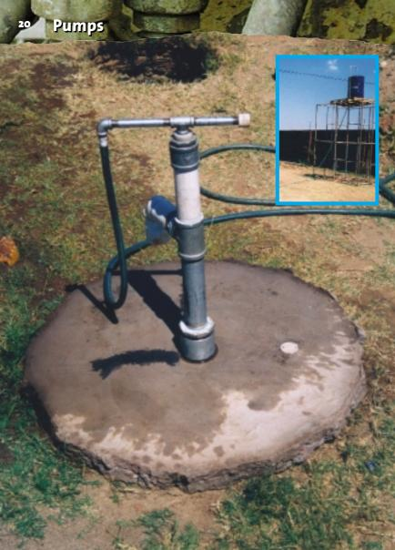
"A complete domestic water system costs US\$ 90, including a 15 m deep well, a PVC pump and a water tank in the kitchen".
