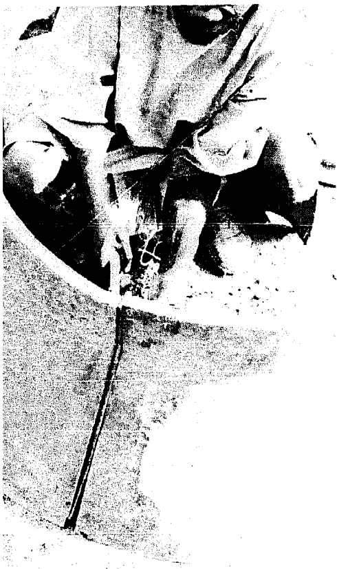
Photo 52 Building Up The Cutting Ring Mould – d) Removeable wedges to loosen sections for removal. – Upper Volta.
