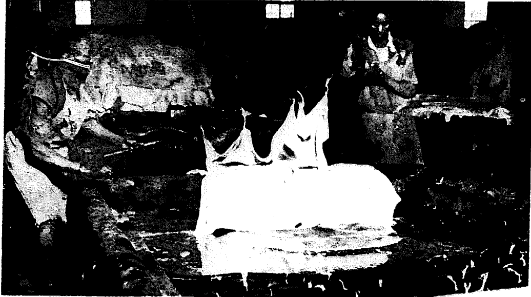
FIGURE 86. - Moving hides in suspender pits.
