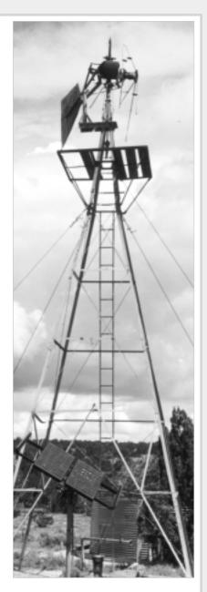
The well under this dead windmill has been brought back to life by a solar submersible pump powered by a 120-watt array.
