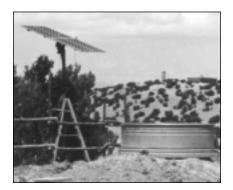
A 300-watt solar array powers a pistontype solar submersible pump located 550 feet deep in a nearby well.
