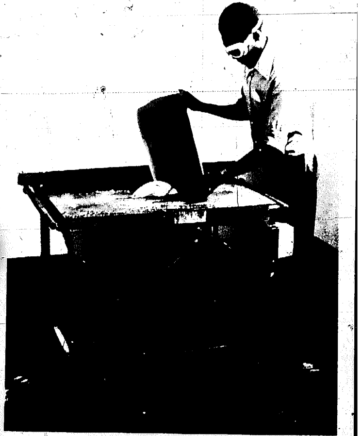
FIGURE 15: Cutting scrap on a circular saw.
