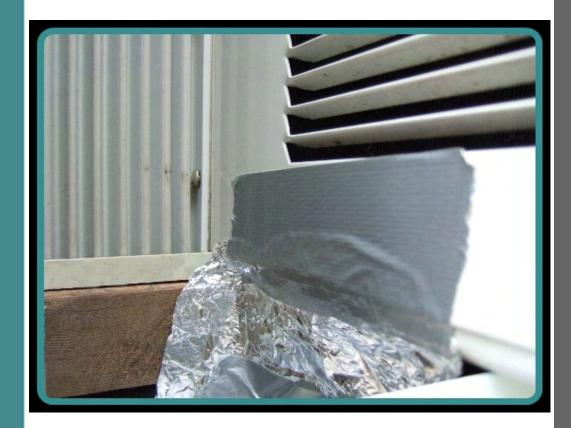
The window a/c unit is sealed at the bottom with aluminum foil and duct tape, to prevent birds from nesting underneath.
