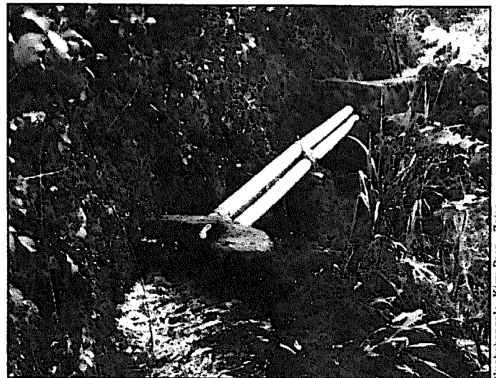
Fig. 5.9. Pipes are used to connect two sections of a canal where a steep, unstable section had to be traversed. Three lengths were used because a single pipe of the necessary diameter was not available.
