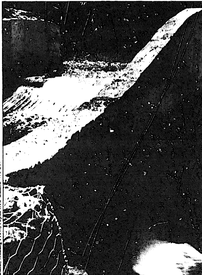
Fig. 5.64. A view of the drop intake shown in Fig. 5.63. Water falling through the trashrack at the upper left can be seen entering the canal at lower right.
