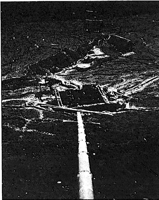
Fig. 10.15. The penstock descends from the forebay to a mill under construction.
