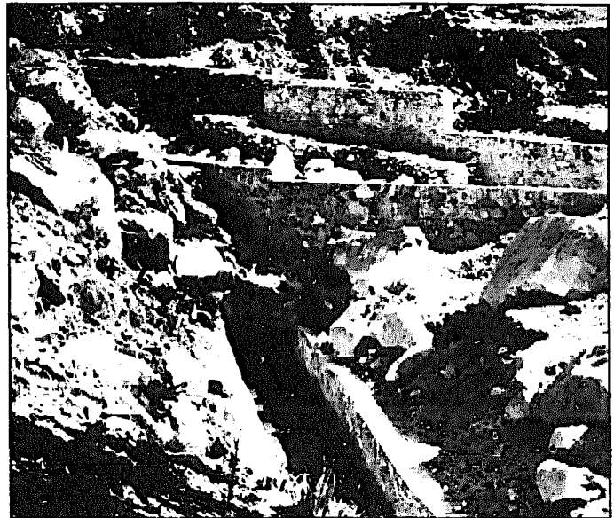
Fig. 5.12. A power canal passes through a culvert under a ravine which collects considerable runoff during the monsoon. Two walls visible above the culvert keep this flow within its banks.
