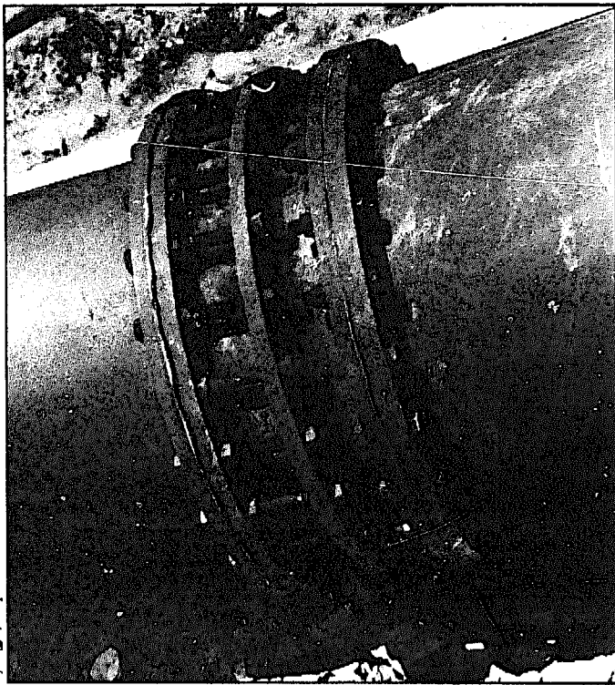
Fig. 5.134. A sliding-type expansion joint.
