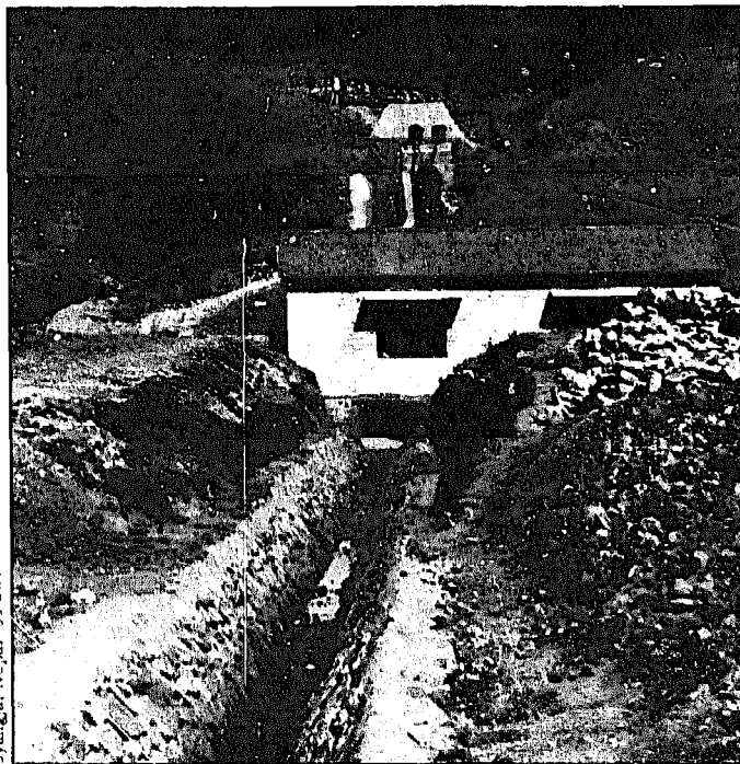
Fig. 5.25. This tailrace will carry water from the powerhouse back to the stream. The short penstock can be seen behind the powerhouse (also see Fig. 5.121).
