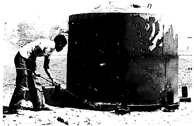
8. Allow the kiln to heat up for 30 to 60 minutes until the bottom section is so hot that it is unpleasant to stand close to the kiln. During this period fill the joints between the main sections of the kiln with sand and place the smoke stacks in position over the support collars of alternate air channels.
