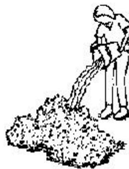
Mix the fine soil with the filler and the water
